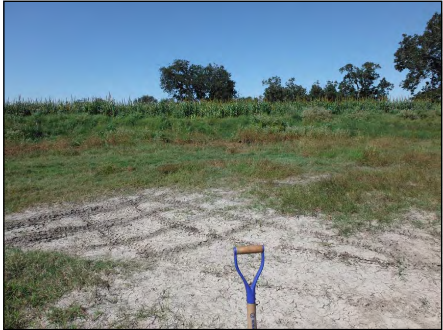
Photo 7: Dike on northwest side of impoundment. View is to the northwest from location of wetland test plot.
